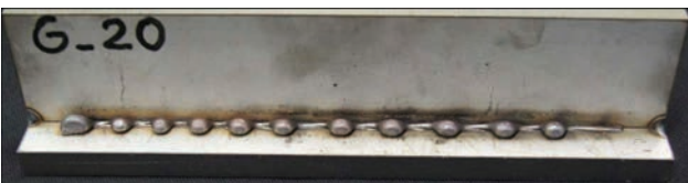
Figure 17. Back side of T-joint of sheets of 20 mm thickness — humps
