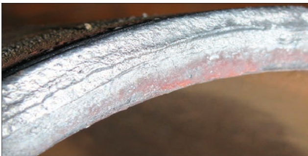
Figure 2. Traces left by welding arc during heating of the outer edges of pipe
