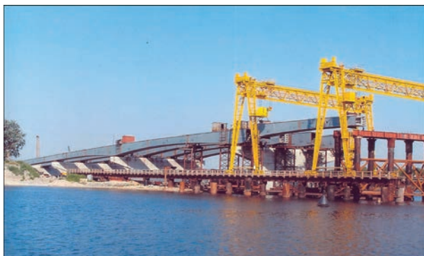
Figure 5. Construction of the Podilskyi Bridge crossing in Kyiv, the arches of which are made of steel 06GBD of the strength class C390
