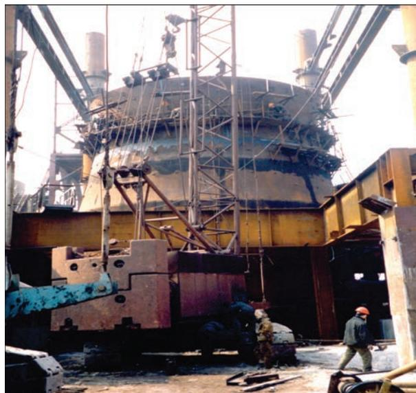
**Figure 7.** Repair of blast furnace DP-2 at the OJSC «Azovstal Steel Plant» using rolled steel 06G2B of the strength class C440
