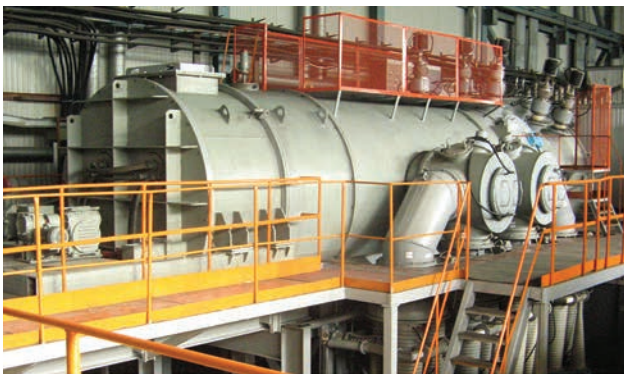
Electron beam installation UE5812
