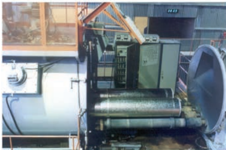
Electron beam installation UE185 for melting the ingot surface
