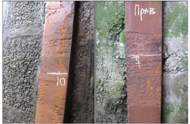
Figure 5. Characteristic damage of working path rails of lift gates in Kaniv navigation lock
