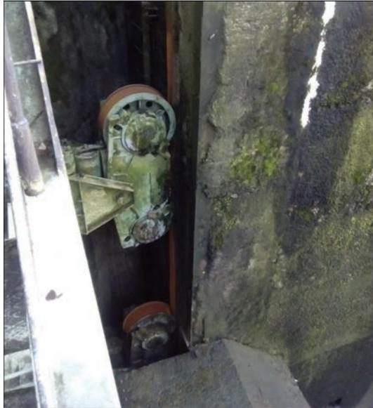
Figure 3. Support carriage of lift gates in Kaniv navigation lock work gates and penstocks is activated by volumetric hydraulic drives.
