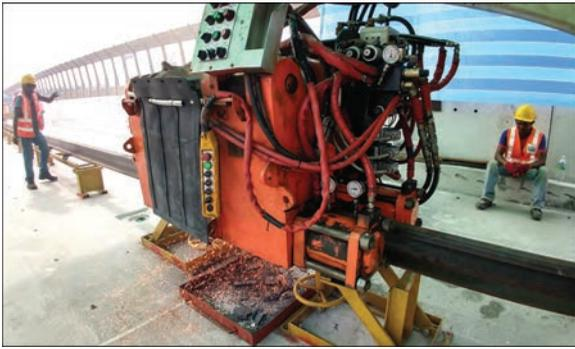
**Figure 1.** Mobile rail welding head K900
