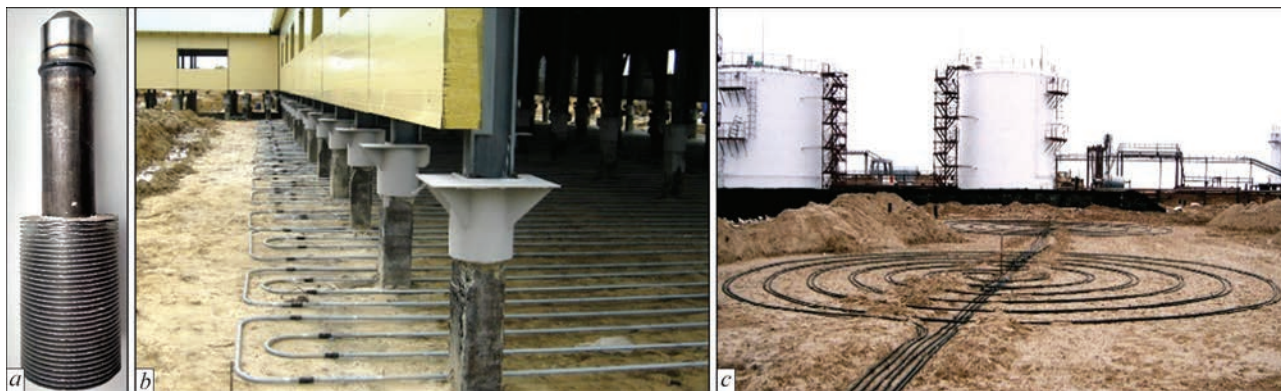
Figure 17. Welding of pipelines for soil thermal stabilization systems, where: a — welded joints of the pipe with the bottom; b — system for soil thermal stabilization: building foundations; c — and oil and gas storage facilities
