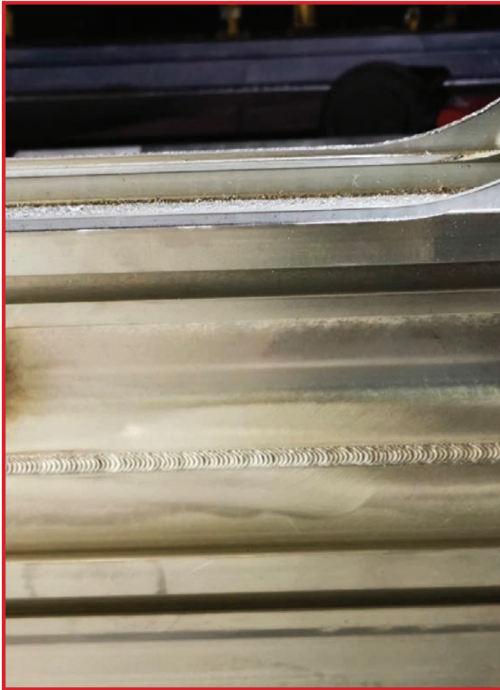
Close-up of aluminum weld showing uniform ripples and clean toe transitions, evaluated per ISO visual inspection criteria
