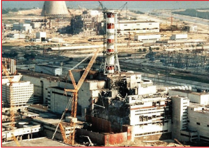
The Chernobyl Nuclear Power Plant after the accident
